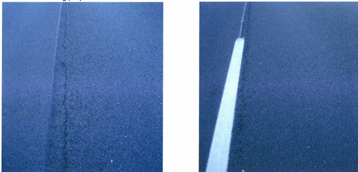
Figura 13: Photos 1 and 2 below demonstrate an open joint as a reflection crack in the asphalt binder layer at the left edge of the 1st traffic lane.
